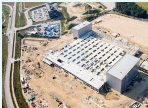
Northvolt Dwa Construction November 2022
